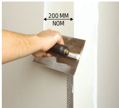
2. Apply first coat to both corner faces
