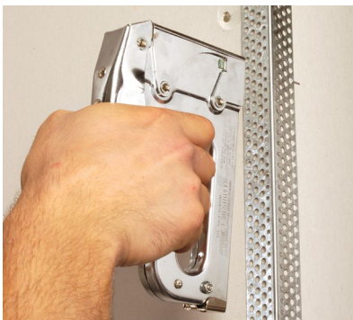
1. Cut angle and fix to sides of corner at 300 mm ctrs
