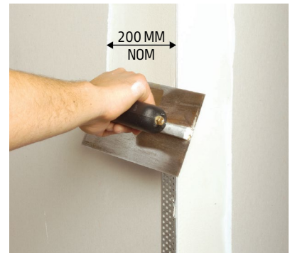
3. Apply second coat to corner faces
