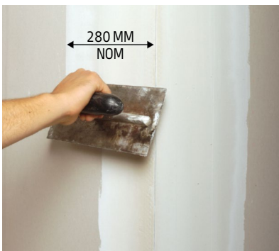
4. Apply third coat to corner faces
